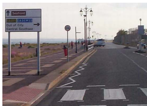
Promenade encroachment - is this good practice? It's a conservation area too.
