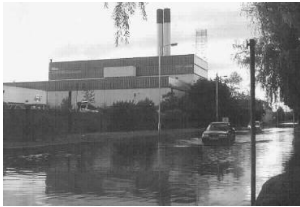
Quartermaine Road in flood
