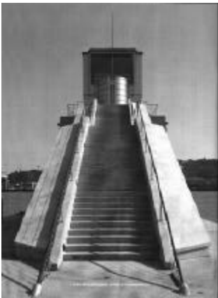
The symbolic lighthouse at Göteborg - a 'think tank', office and ferry service base.
